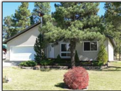
H41 THE BROWN HOME -- With 3 Bdrms, 2 Baths, Approx 1500 Sqft, 2 Story, On Approx .23 Acres, Built In 1997. Save Money On Utilities W/This Energy Efficient/Low Maintenance Home. Tall Pines, Home Water Filter, Air Lock Entry, Berber Carpet, Trex Deck & More. >On Mosswood Dr 167 (brown-his) (313612)
